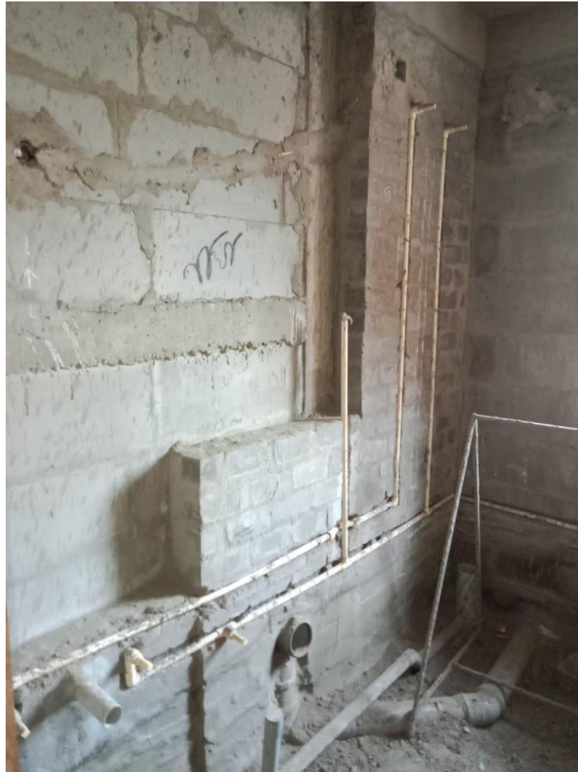
Wing 1: Plumbing work
